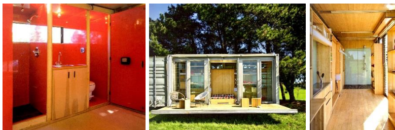
Figure 25: Mobile Units with Certain Facilities
